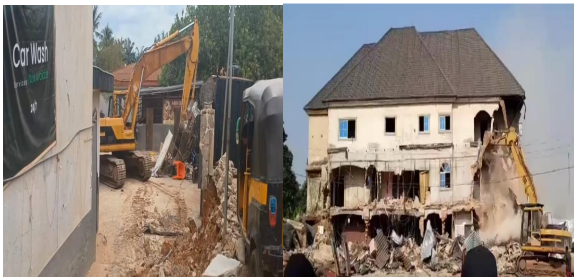
Fig 3: Demolished Hotels (Udoka Golden Point Hotel and Suites, and Airtight Guest House and Bar)
