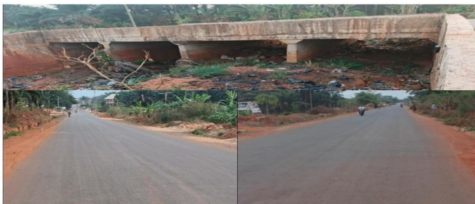
Fig vii: A double view of a newly constructed road and bridge at MCC road Alor-uno gully site
