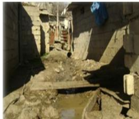
Fig 4: Interior of Djaballah's slum
